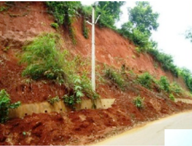
Slope before plantation
